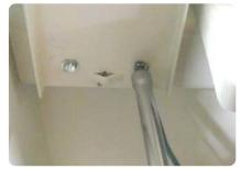
Make certain that the star washer is pinched between the electrical raceway and the terminal on the grounding wire. Star washer should break the paint surface when tightened.
