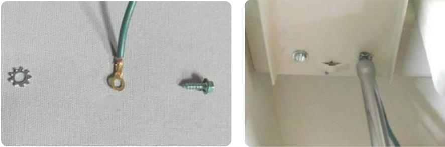
Make certain that the star washer is pinched between the electrical raceway and the terminal on the grounding wire. Star washer should break the paint surface when tightened.
