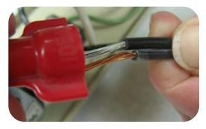
Place a piece of electrical tape around the ends of the black wires from the pilot light and electrical outlet (& spotlight, if applicable) to the 7" black wires on right post. Connect by twisting on wire nut.
